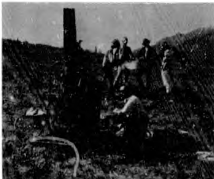
This photograph shows Cantwell resident Mike Pedro operating a steam jenny to thaw holes in the permafrost for fence posts.
