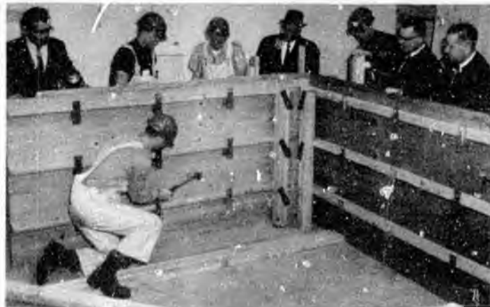
Concrete wall forms erected by apprentices as part of their related training.
