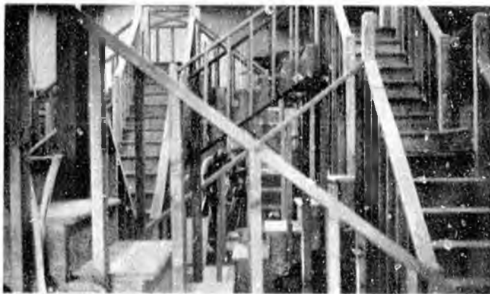
This stair project is an example of work performed by Apprentices in this Program.
