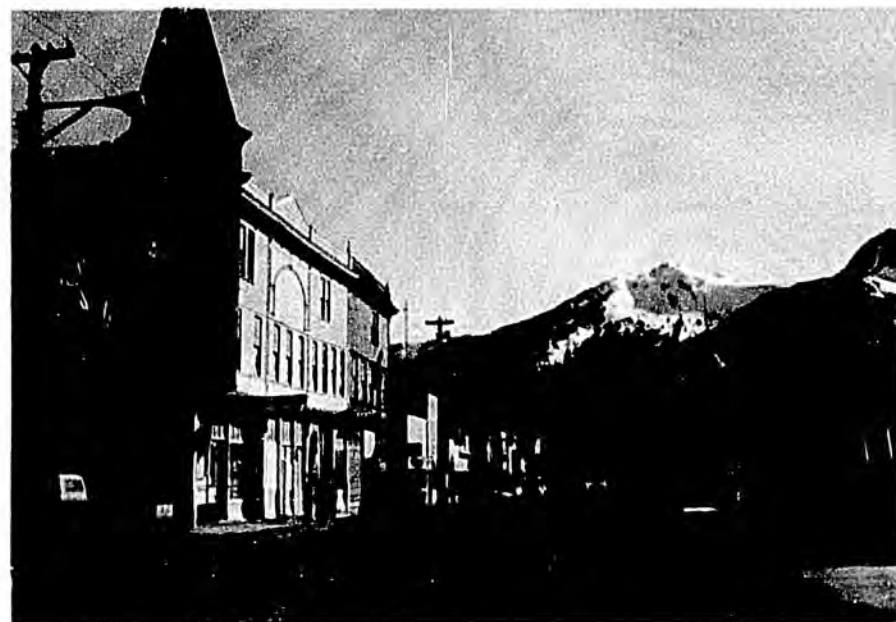
Historic Broadway, Skagway's main street, is preserved today in the historic district of recently established Klondike-Goldrush National Historical Park [O-045]. The quaint false-fronted buildings and wooden sidewalks are visible reminders of the town's once fabled position as the supply gateway to the Klondike Gold Rush. Be certain to visit the Interpretive Center of the National Park Service in the former White Pass & Yukon Route railroad station building at the foot of Broadway.
