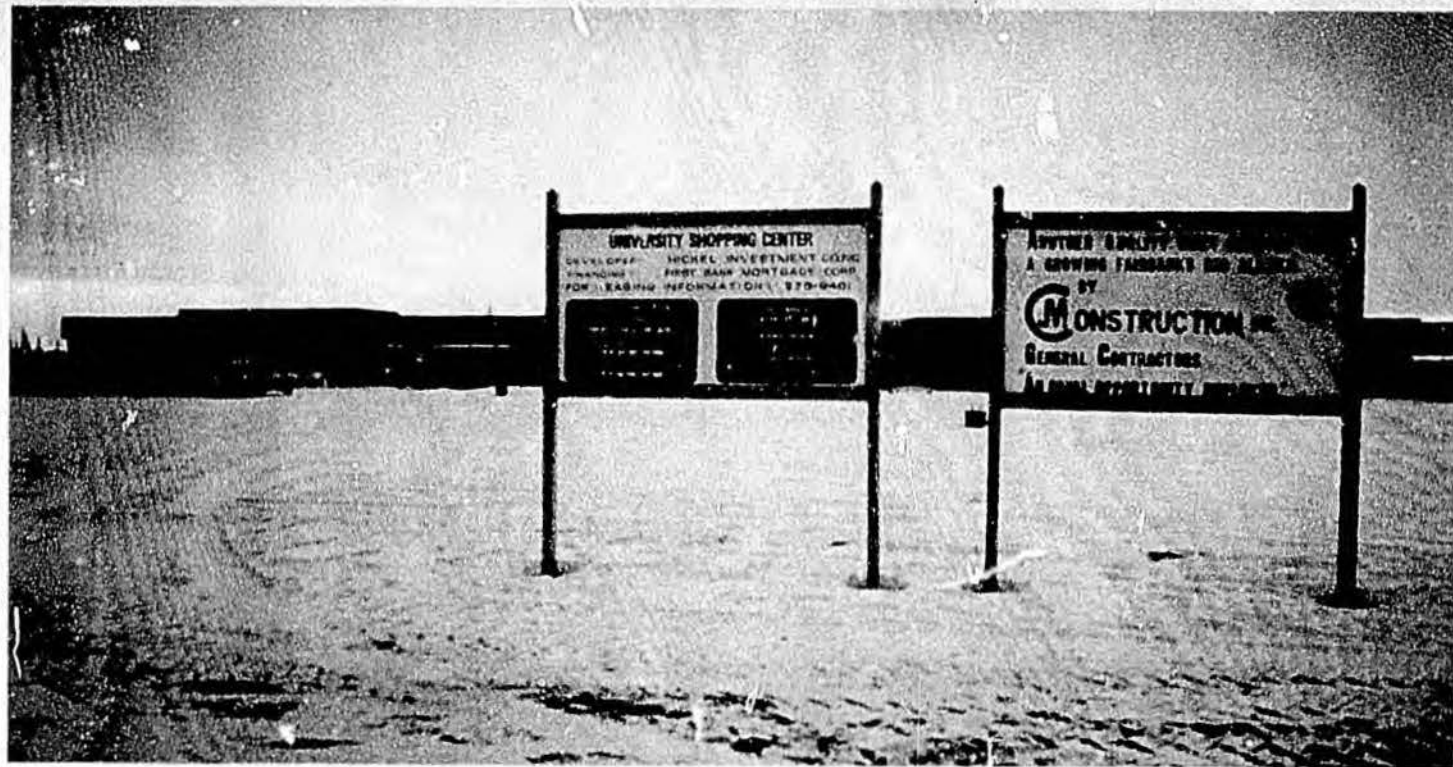
HICKEL MALL —A mall addition to the Safeway store on Airport and University is expected to be open for leasing in spring
