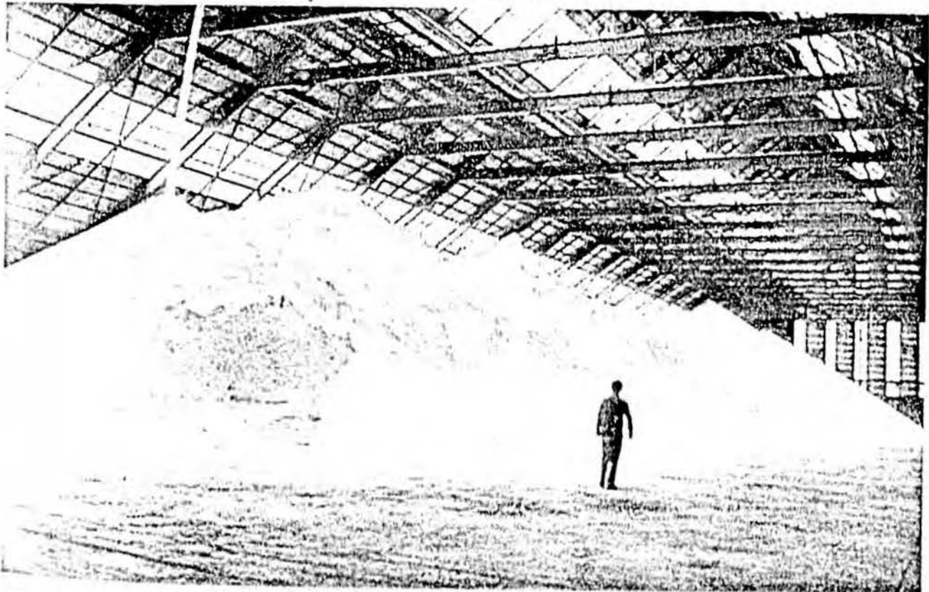
Petrochemical project in the Republic of Korea. The Hankook Caprolactam Corporation's plant has now begun production.
