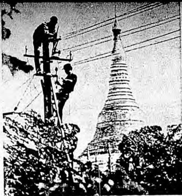
Work proceeds on the Power Transmission Project in Burma.
