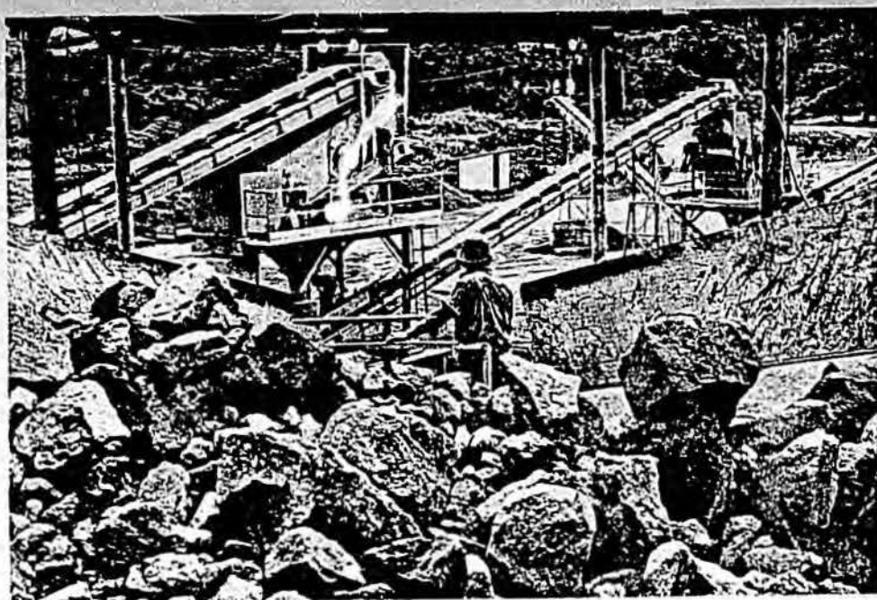
RAW ROCK MATERIAL SLIDES DOWN chute of this bulldozer-scoop to concrete mixer producing materials for rebuilding Managua largely destroyed by 1972 earthquake. The enterprise expanded operations with credit from the Inter-American Bank provided to the Banco Nacional de Nicaragua following the disaster.
