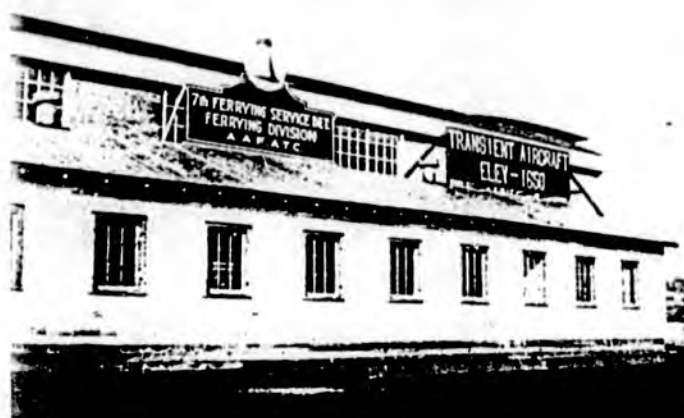
Operations building at the Bismarck, North Dakota, detachment. COURTESY 7th FERRYING GROUP ASSOCIATION
