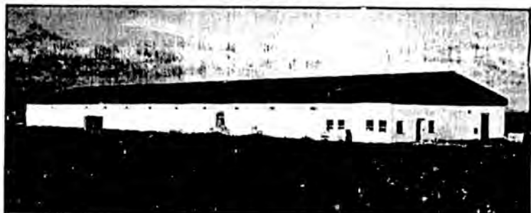
The hatchery building at Islandsfax.
