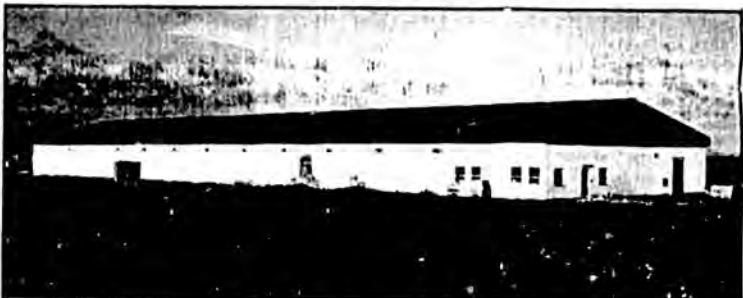
The hatchery building at Islandsfax.
