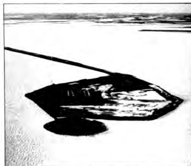
Camp construction on the Main Production Island (MPI), foreground, will begin in March of next year, and installation of two permanent bridges on the causeway will be completed in April.
