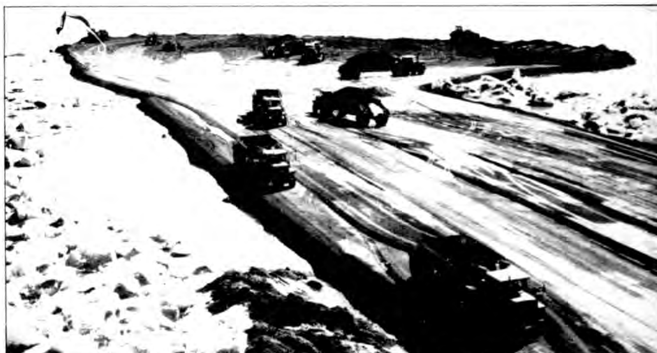
Requiring about 6.5 million cubic yards of gravel, this first phase of Sohio's Endicott Project was the largest project of its kind ever conducted on the North Slope.
