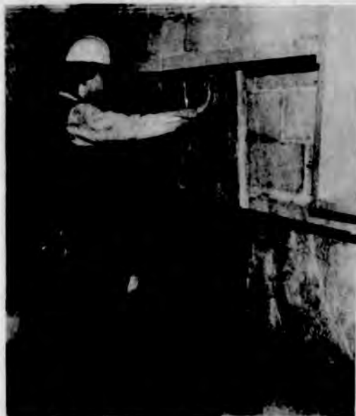
Insulation contracting is an important element of the Rhode Island energy conservation program.
