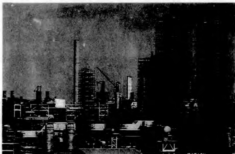
BP/ICI cracker at Teesside under construction
