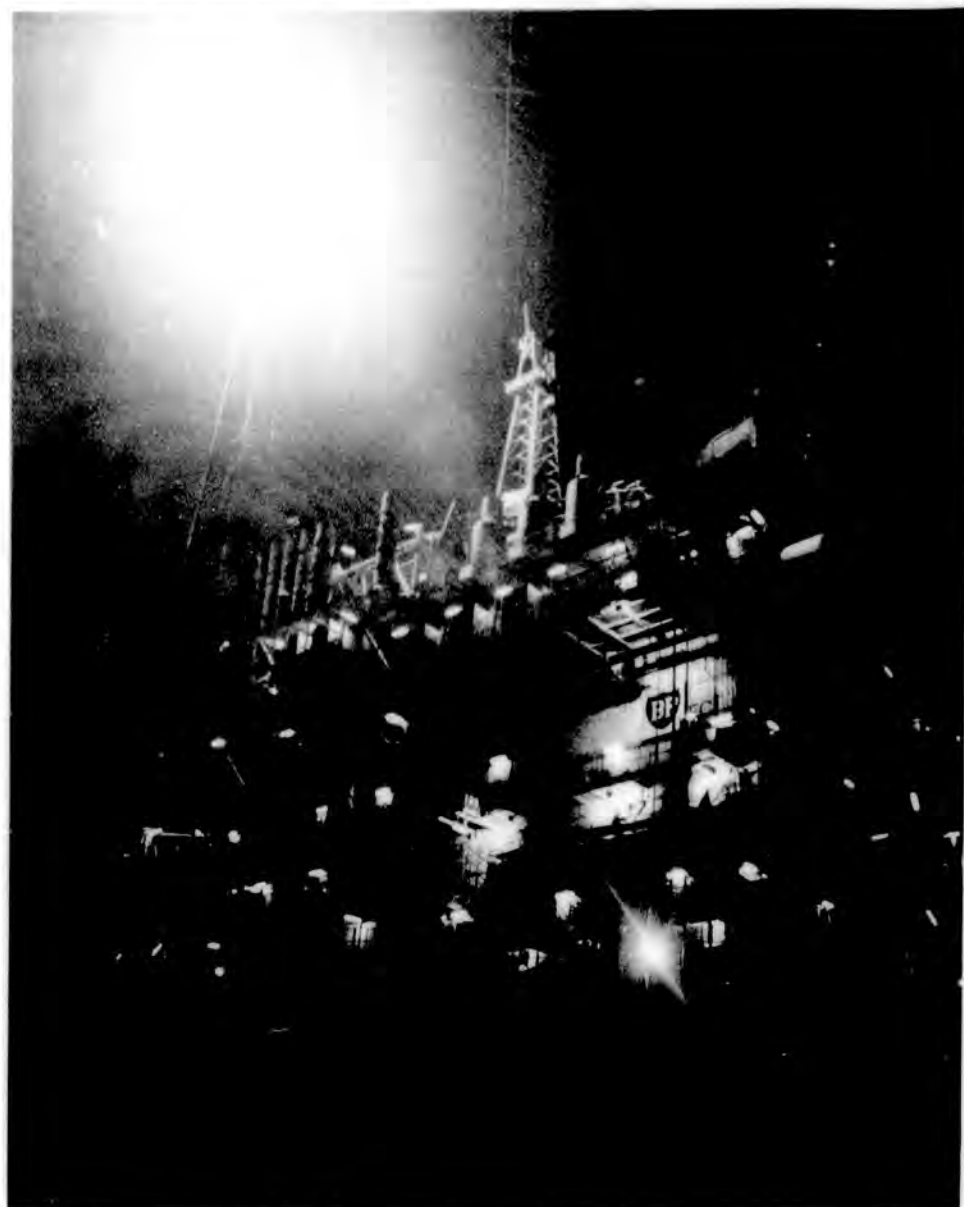
Production platform in the North Sea
