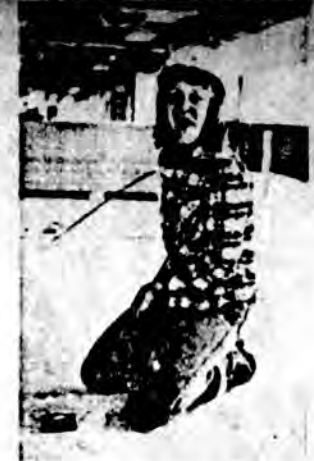
Cynthia Thomas, an 80 per cent apprentice of Local I.B.E.W. 1547 is caught in the act of stringing electrical wire.
