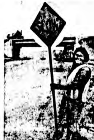
Frances Greenway of Fairbanks Labors Local 942 makes sure safety is ensured on the new Steese Highway project.
