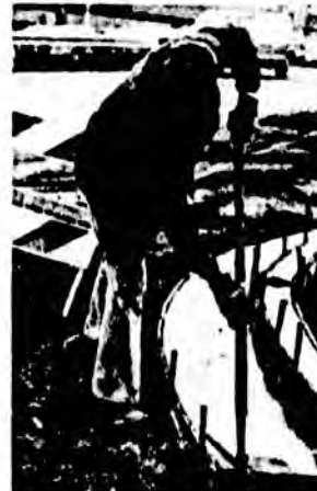
This cement form gets its final touches from John Jackson of Plasterers and Cement Masons Local 867.
