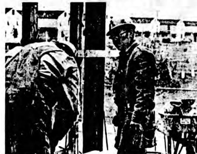
David Victoroff works on cement forms for Baugh Construction. He is a member of Local Carpenters Union 1281.
