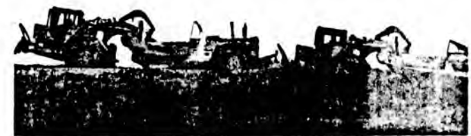
Northwestern Construction, Inc. scrapers working to level the earth for the new runway addition at Anchorage International Airport.
