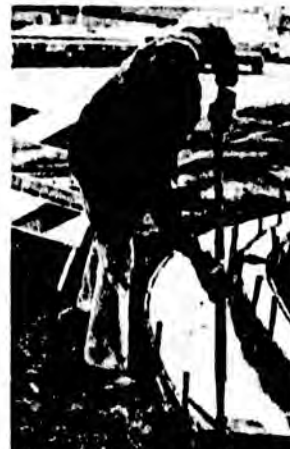
This cement form gets its final touches from John Jackson of Plasterers and Cement Masons Local 887.
