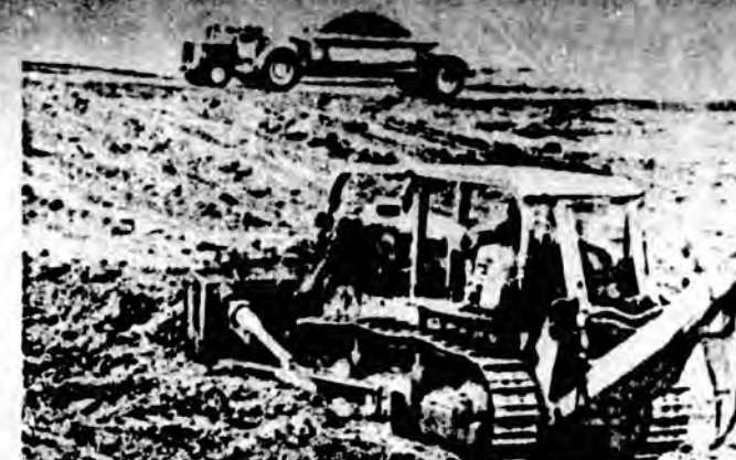
A Moose Creek dam gravel pit gets cleaned out for future recreational use. The sides will be covered with top soil to encourage natural plant growth.
