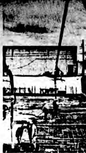
Ken Brady Construction Company's crew working on Alaska's largest single concrete pour ever made. It will be the main foundation of the new International Brotherhood of Electrical Workers Trust Tower.
