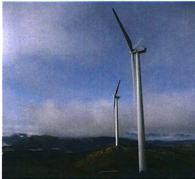
Kodiak Electric Association installed three 1.5 MW wind turbines on Pillar Mountain in 2009 and then doubled the size of the wind farm in 2012. The project now supplies more than 18% of the community's electricity. Combined with the Terror Lake hydroelectric project, KEA can shut off their diesel generators almost all year.
