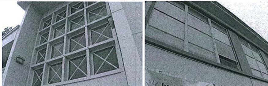
Figure 2: View of Single Pane Windows and North Facing Windows
