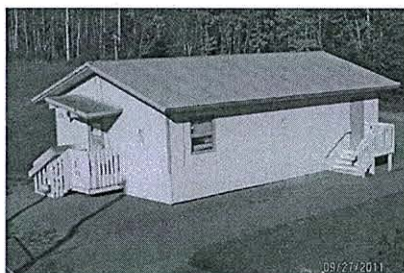
Figure 1: View of Chinook Elementary Relocatable Classroom
