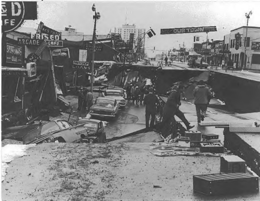
4th Avenue After Earthquake
