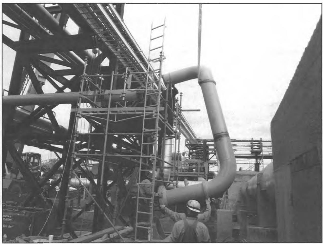
Recirculation pipe installation at PS4
