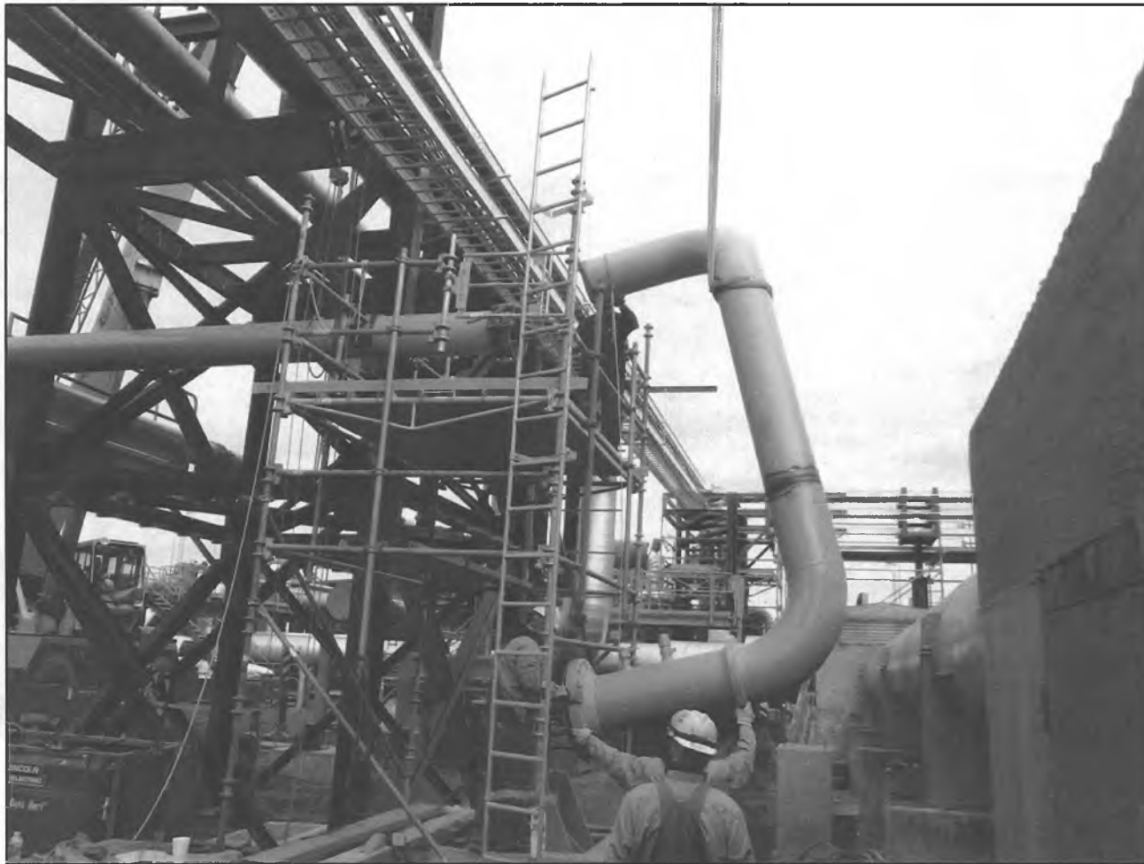
Recirculation pipe installation at PS4
