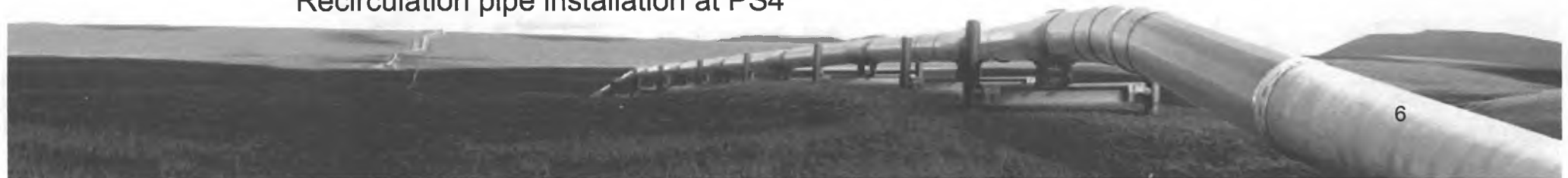
Recirculation pipe installation at PS4
