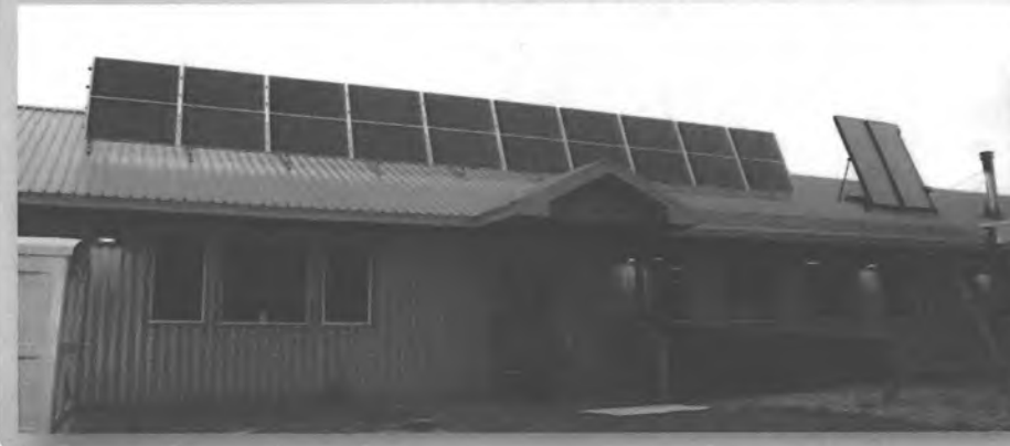
Solar Install Nenana Teen Rec Center
