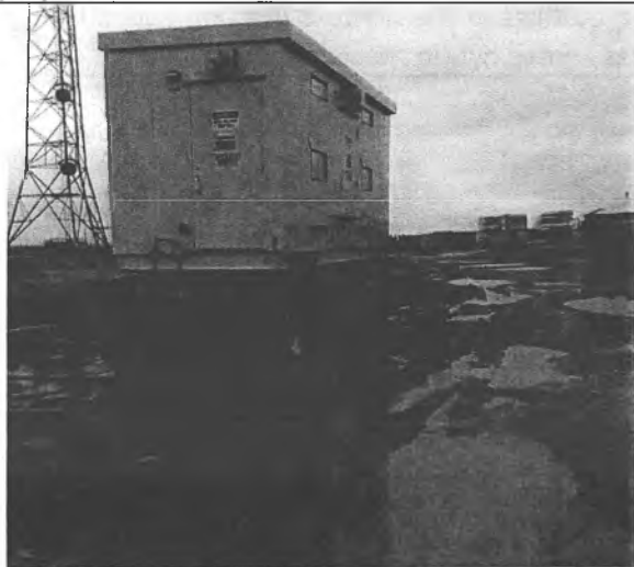
Battery and enclosure awaiting freeze up
