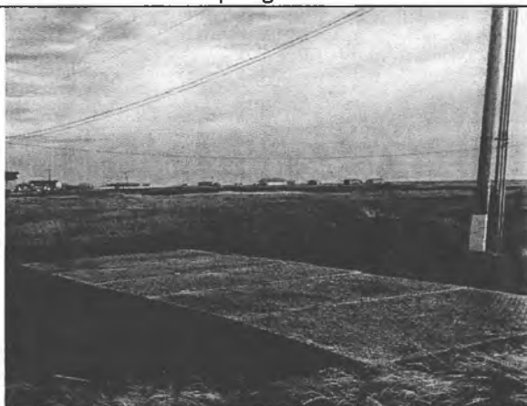
Site mats positioned awaiting the battery
