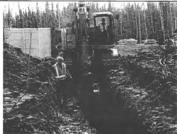
Digging the trench for the coil
