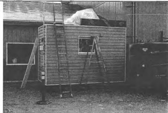
Testing box under construction
