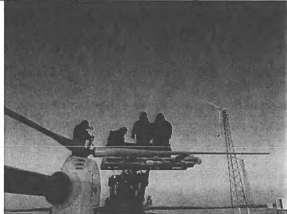
Installing turbine blades
