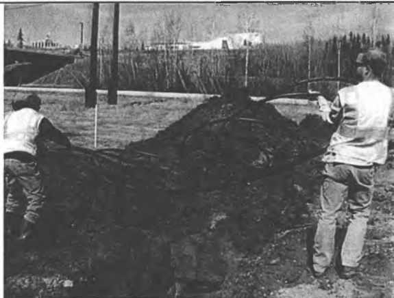
Installation of the slinky loop
