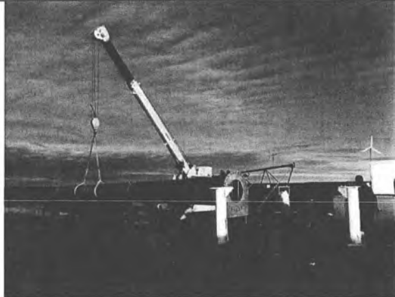
Assembling the tower
