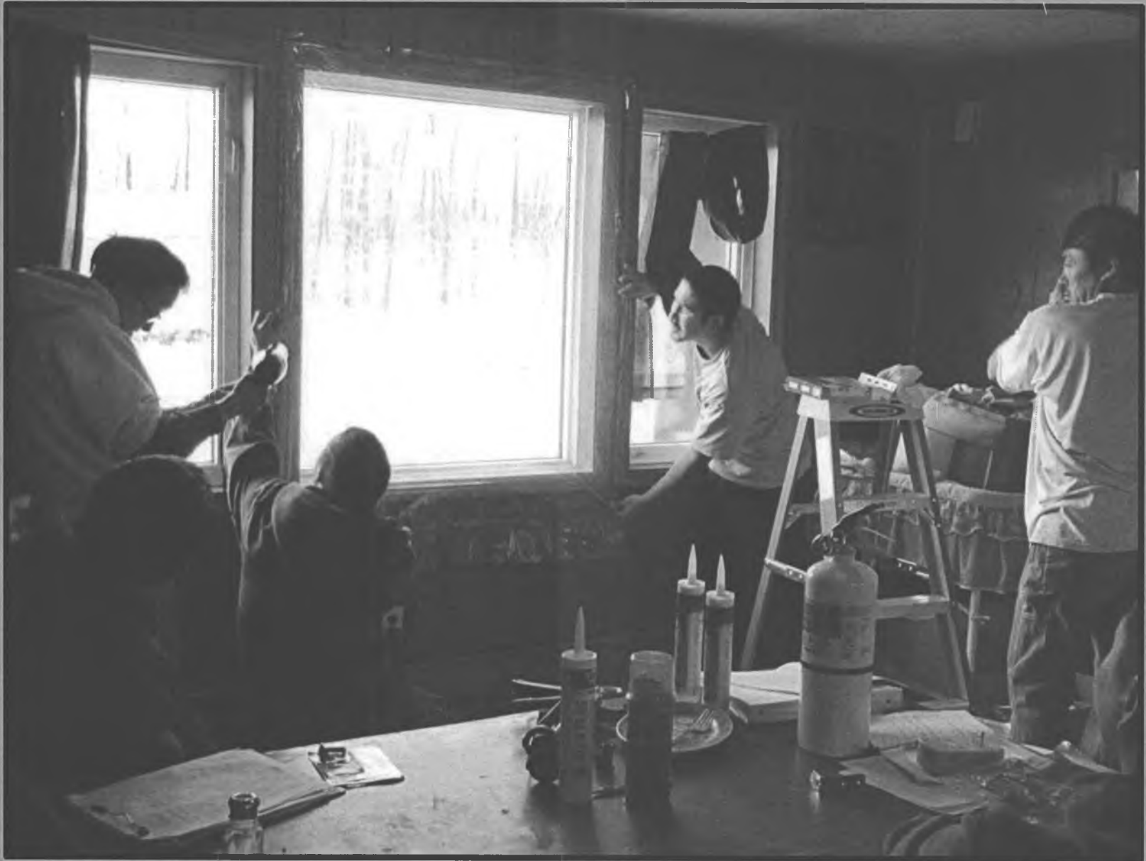
Crew Leaders Teach Crews and Practice Installation
