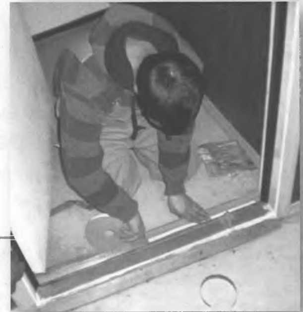
Installing door sweep and weather- stripping
