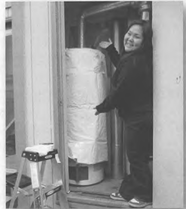
Installing water heater blankets and teaching maintenance
