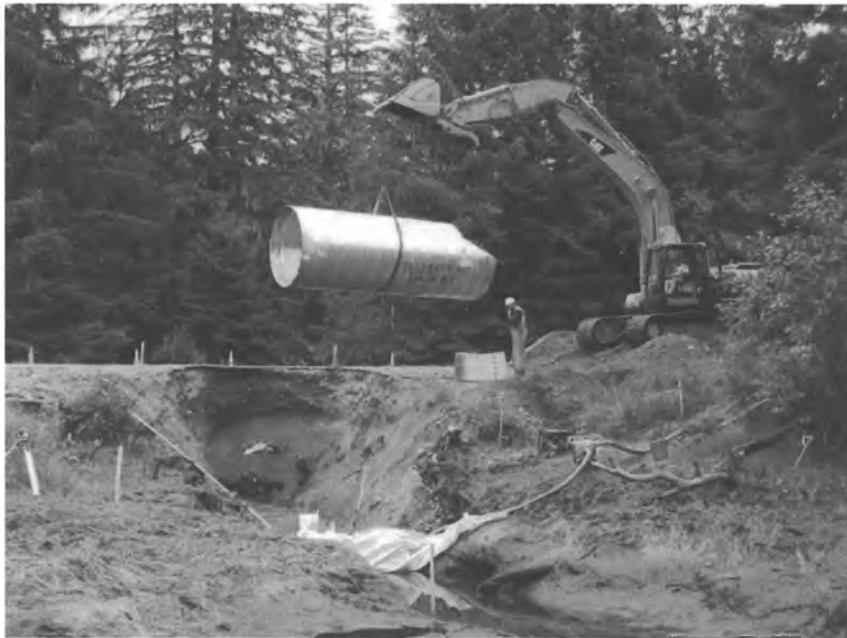
Culvert Installation
