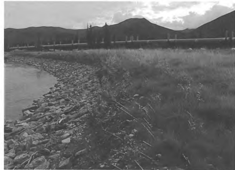
Stream revetment and pipeline
