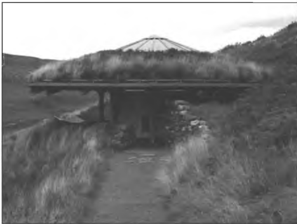
This trailhead structure in Knochan Crag National Nature Reserve, Scotland, harmonizes with the stone and heather of this mountain environment.
