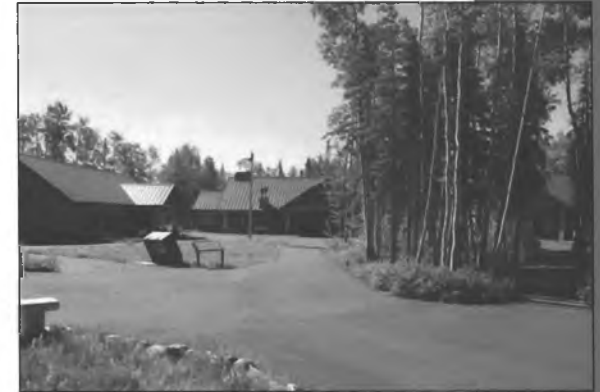
Wrangell-St. Elias National Park used a campus concept for their visitor center development, with separate buildings for the information center, exhibits, meeting room, and restrooms. This is an alternative that could be considered for the transportation hub.
