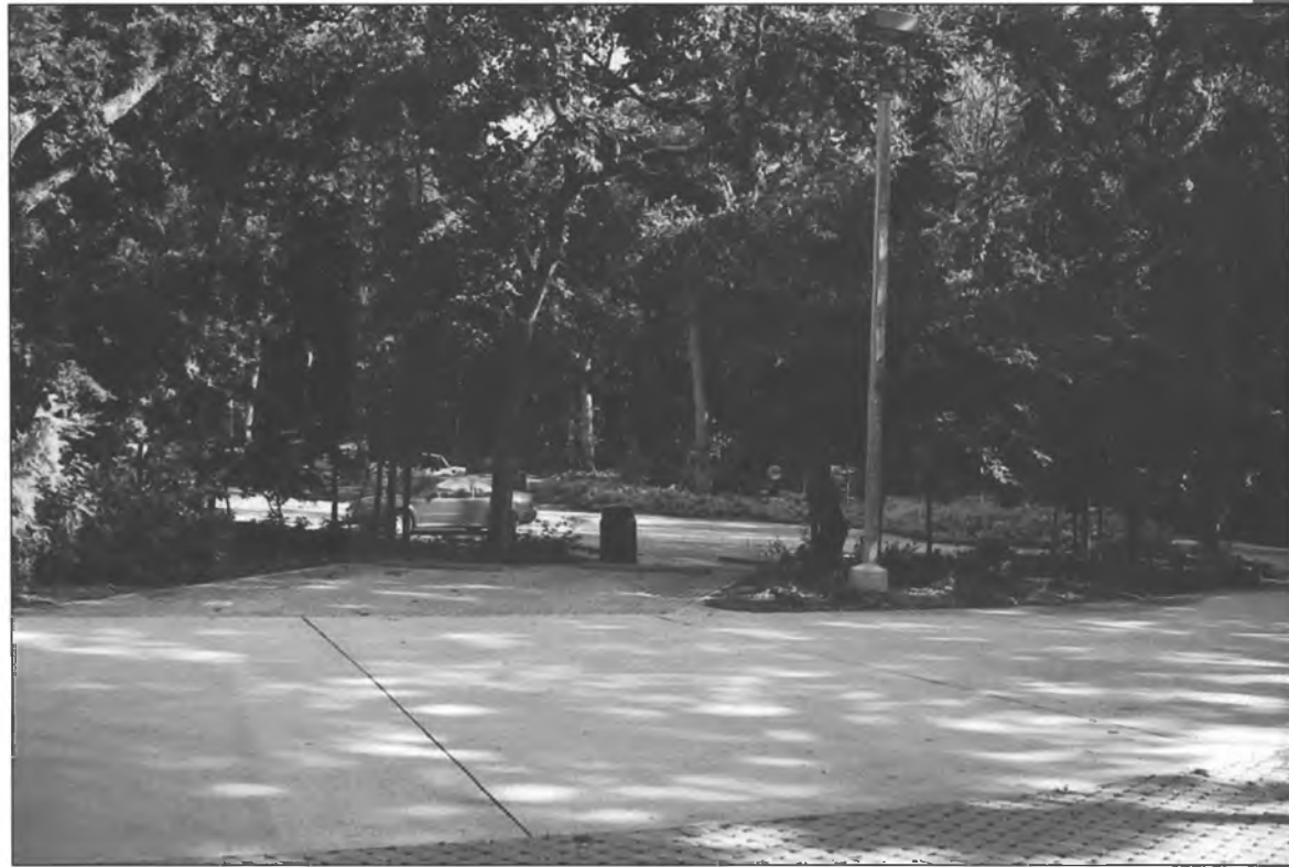
To minimize physical and visual impact, parking lots should be buffered with vegetation and incorporate porous parking surfaces, like this one at the River Legacy Living Science Center in Arlington, Texas.
