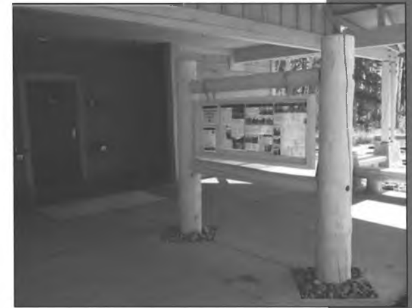
The restroom entrances at Wrangell-St. Elias National Park include a bulletin board, roofed seating, and drinking fountains.
