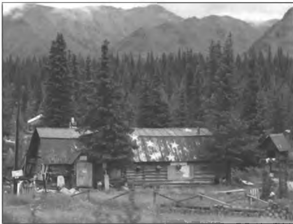
Homesteads in Alaska are creatively constructed of locally available materials. This cabin showcases rough log construction, a metal roof, and a traditional cache. August, 2007
