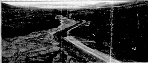
2007 Dalton Highway: Grade heightening at MP 241 to 242 to alleviate snow drifting, and aufeis.
