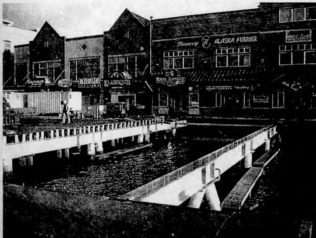
Ketchikan Dock Replacement
