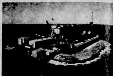
Northstar's production facilities were built in Alaska and sea lifted to the North Slope.
