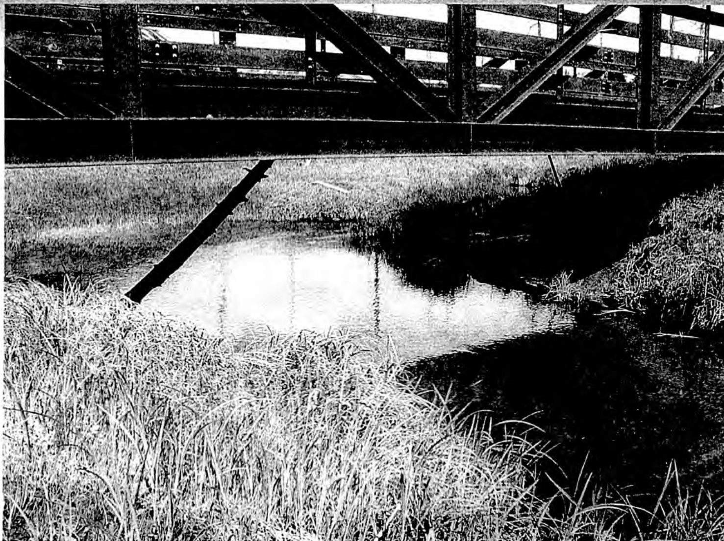
Multi-use trail bridge, Tidewater Slough, Girdwood , Alaska
