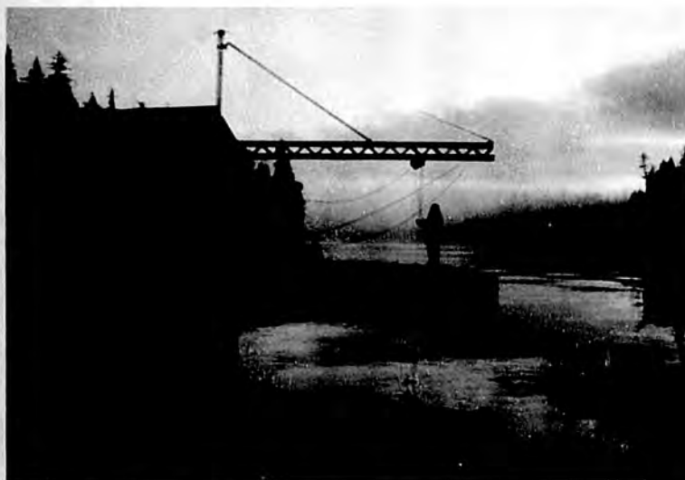
Floating oyster processing facility on Prince of Wales Island
