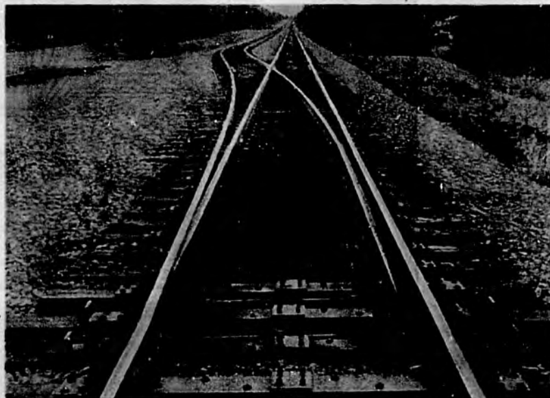
Sidings, such as the Pittman Siding constructed in 2001 pictured above, allow trains traveling in opposite directions on the main track to pass.
