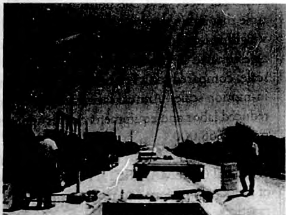
The pictured installation in the Lower 48 demonstrates how the heavy weigh bridge requires use of a crane to set the structure in place upon the concrete foundation.
