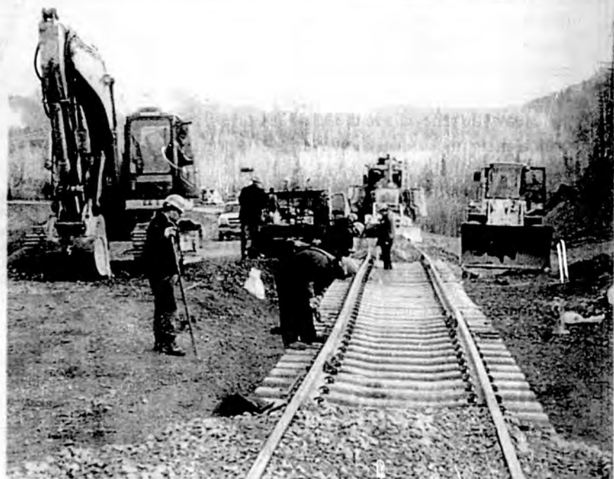
An Alaska Railroad crew installs new track that is improved with continuously welded rail and concrete ties.
