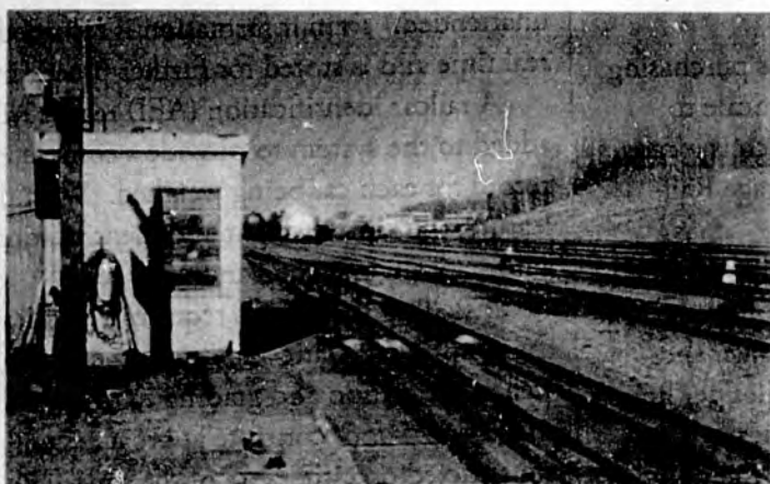
The existing old static scale is located in the northeast area of the Anchorage Rail Yard. The new weigh-in-motion scale will be installed in this same location.
