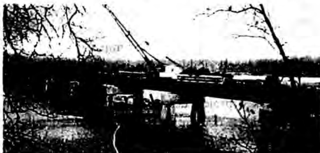
At Knik River Bridge (MP 146.1) new piers and a new south span were constructed in 2005-2006. Demolition of existing piers is scheduled to be complete in 2007.
