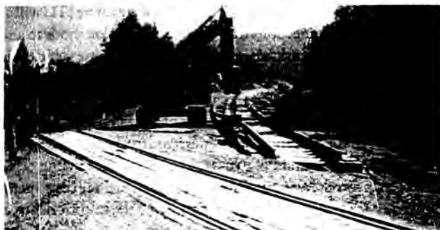
Intersection of new and old alignments at MP 126, near the end of the realignment on Fort Richardson.
