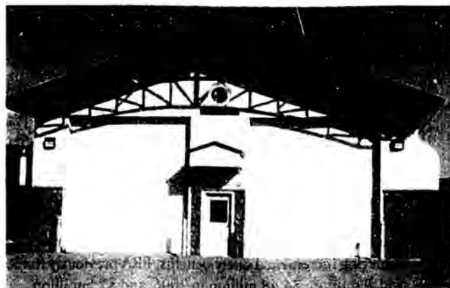
The first Section Maintenance Facility was built in Cantwell in 2006.
