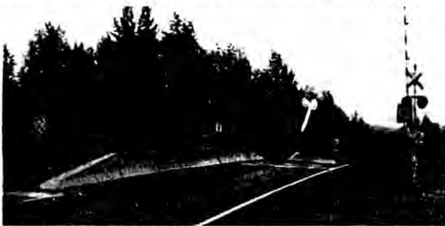
A median barrier is installed at an Anchorage crossing.
