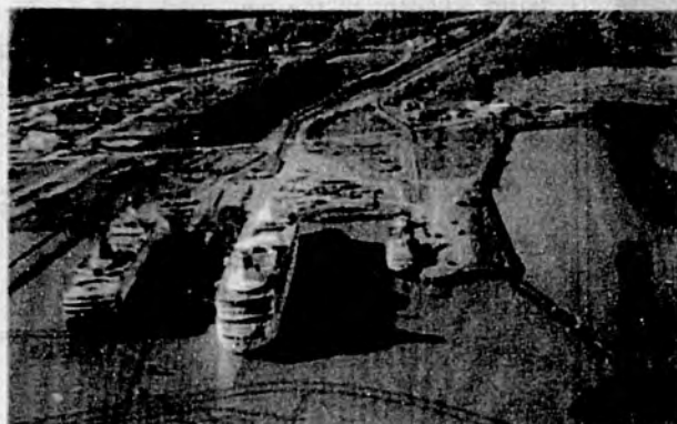
The refurbished passenger dock, left, and the freight dock, right.
