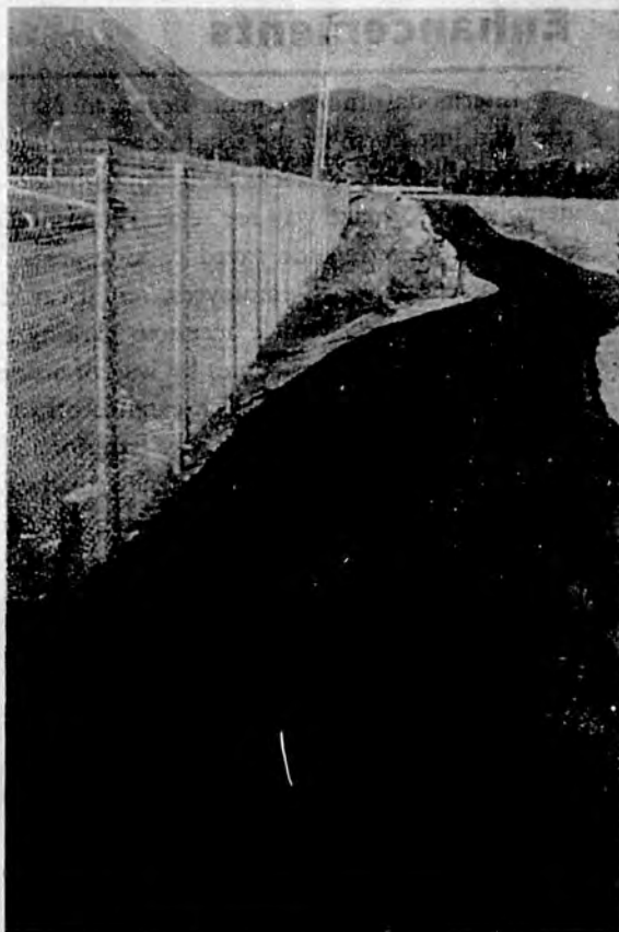
New security fencing is installed.
