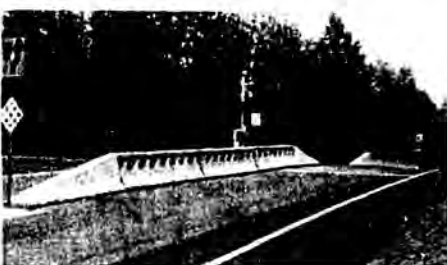
Median barriers at Oceanview crossing.
