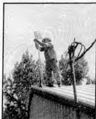
Mac Dearman installs a wireless access point. (see p. 21)
