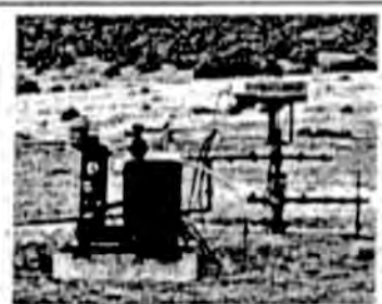
Water Pump and gas Engine
