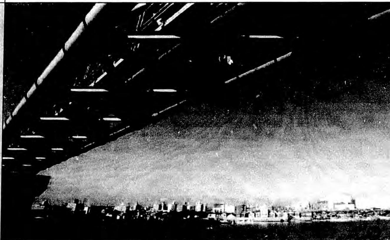
December 1999 saw the completion of the Keihin and Yokohama transmission pipelines. Tokyo Gas now boasts a 300km-long supply loop encircling the greater Tokyo area. Pictured is the Tsurumi River Bridge, which was built for the Keihin Transmission Pipeline.
