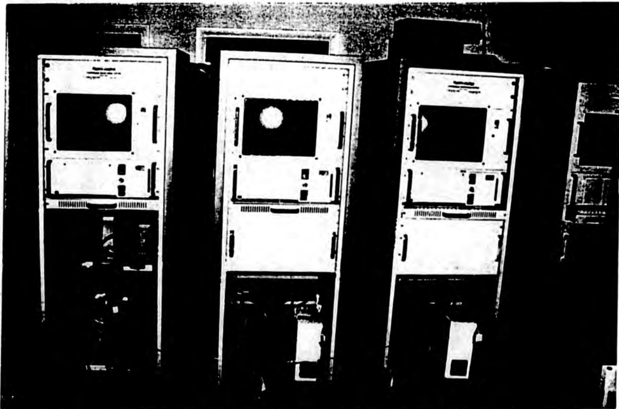
Accelerometer computers used for the TAPS Earthquake Monitoring System. (See p. 33)
