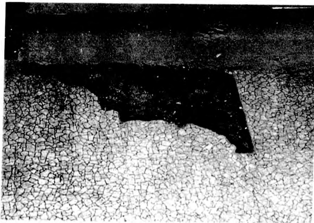
Damaged Floor Tile and Mastic
