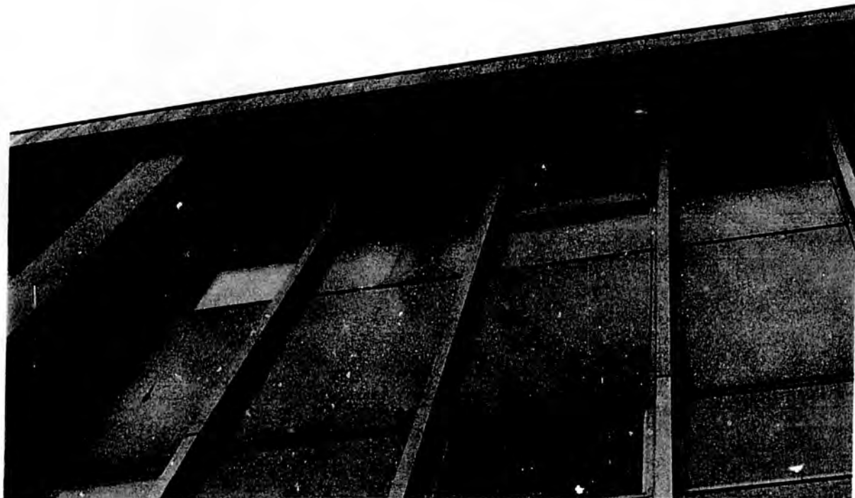
Delaminating Exterior Panels
