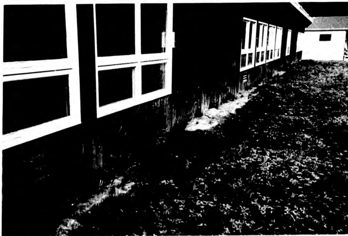
FOUNDATION DAMAGE: Vegetation is growing in the cracks of the foundation. Water leaks through these foundation cracks into the building.
