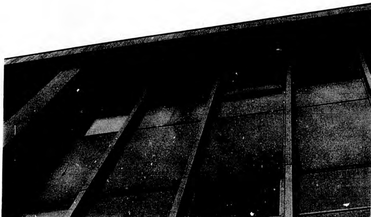
Delaminating Exterior Panels
