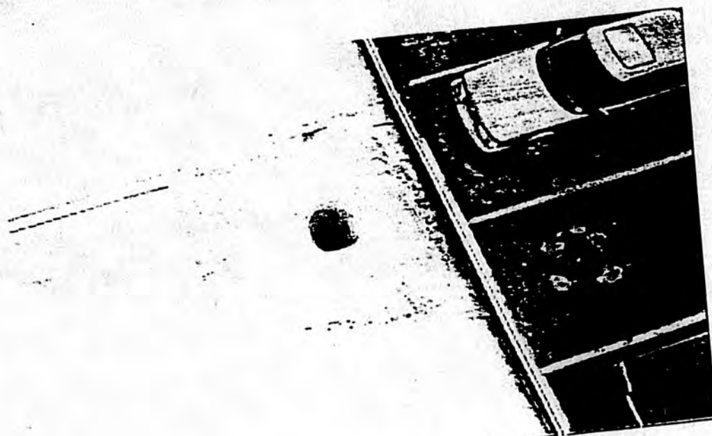
Figure 9 Main building roof drain ties into old roof interior gutter
