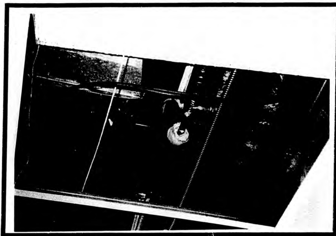
Description of Photo: Friable asbestos, north hallway ceiling, 3rd floor.
