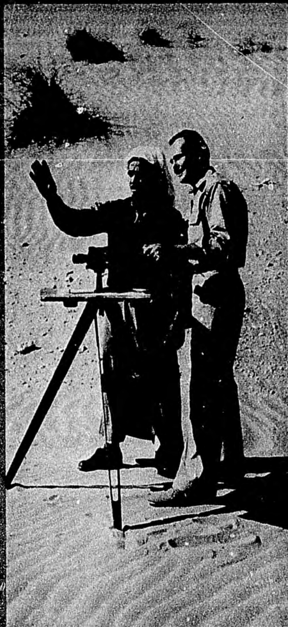
CONSTRUCTION of pipeline and production facilities has picked up in Saudi Arabia as nation pushes for new highs in oil output.
