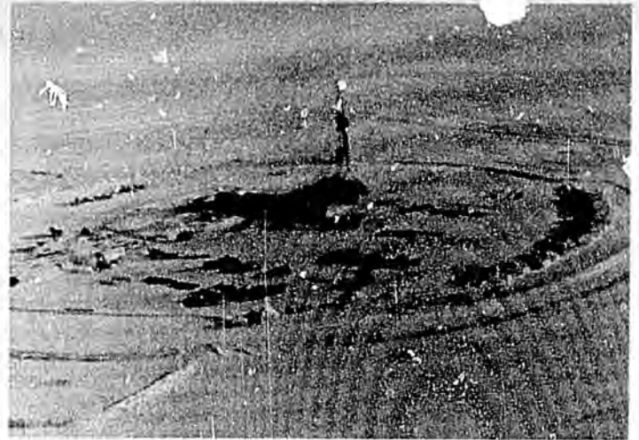
Union Oil's East Harrison Bay Ice Island near Thetis Island was the first man-made offshore structure in the U.S. Beaufort Sea. The well was plugged and the island melted in 1977. Union has not revealed the results of the exploration. The proposed EXXON experimental ice island would be larger, designed to survive annual breakup.
