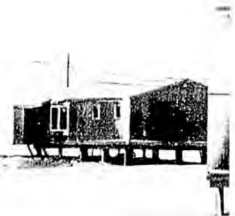
HOMES CONSTRUCTED BY BNC CONSTRUCTION Company for the Association of Village Council Presidents' Housing Authority in Bethel. Supplier was Bethel's Guinn Lumber Co.
