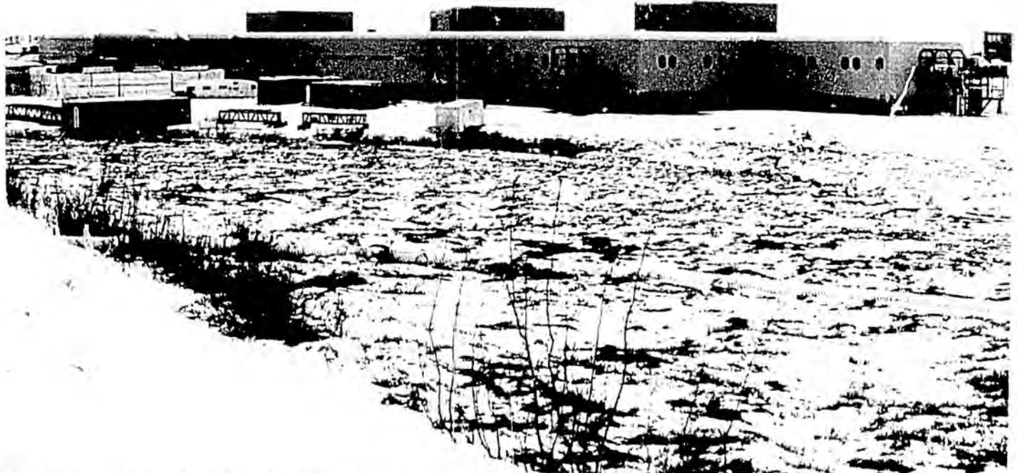
NEW PUBLIC HEALTH SERVICE HOSPITAL currently being completed in Bethel by Hoffman Construction Company. The $30 million structure is mounted on some 350 steel pilings. The 94,000 square foot hospital is one of the many construction projects underway in the Delta area.
