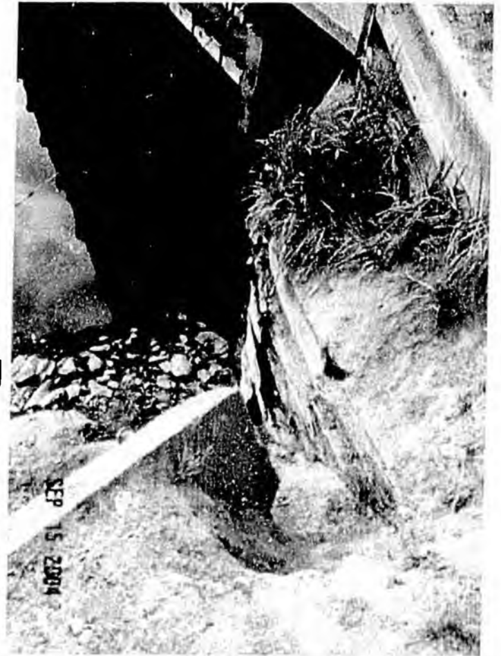
Damaged Piles from Ice Flows
