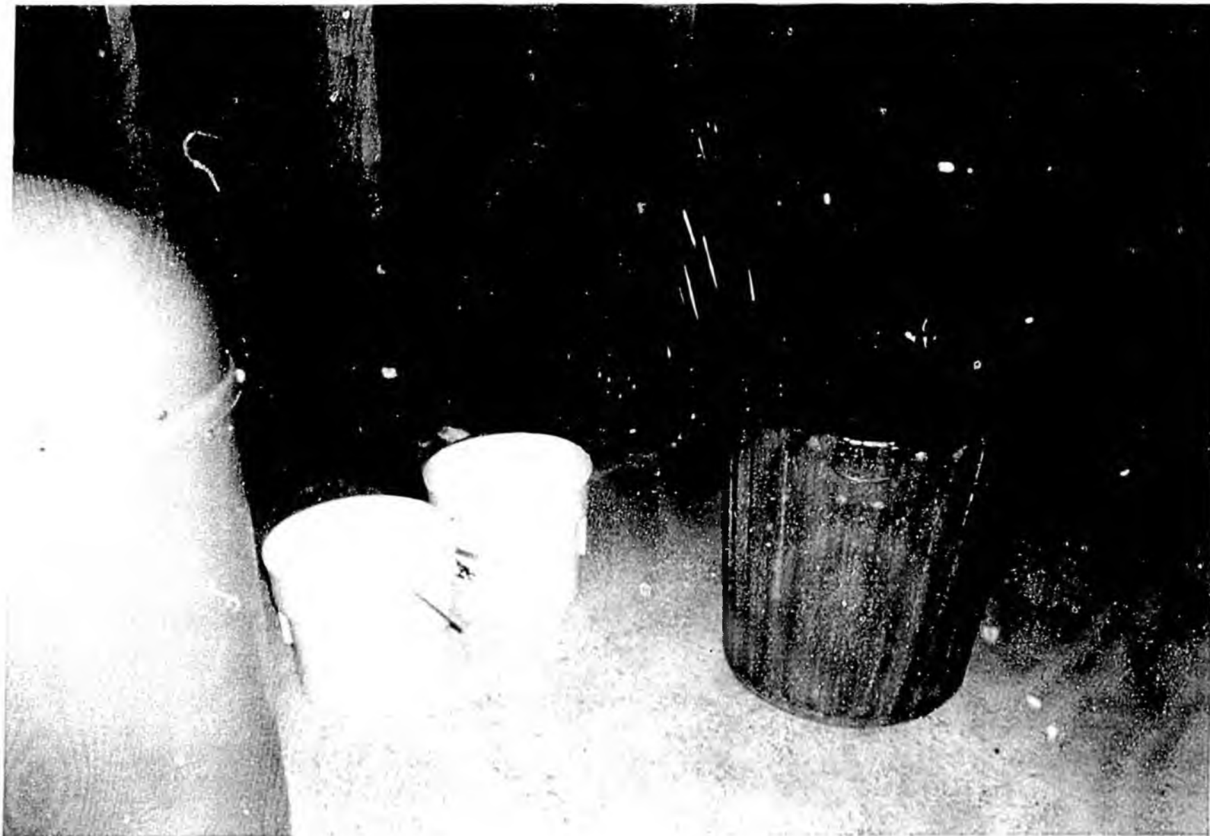
Existing roof leaks at Sitka Pioneer Home – South Wing
