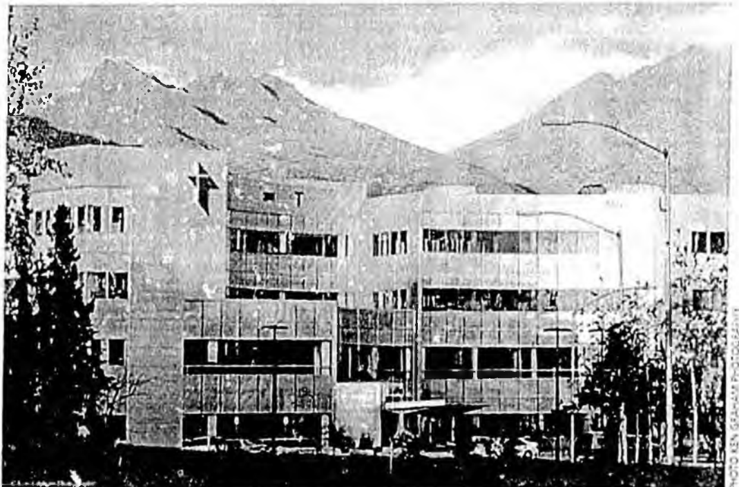
Providence Hospital addition, Anchorage
