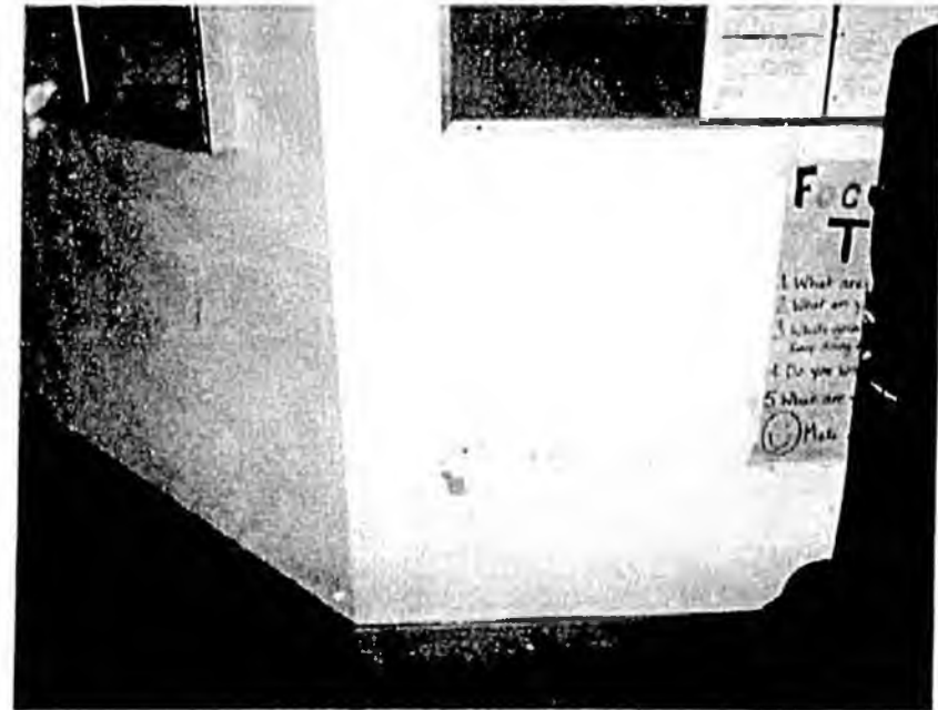
Priority 15: Fahrenkamp Center Wall Protection ($24,700)
