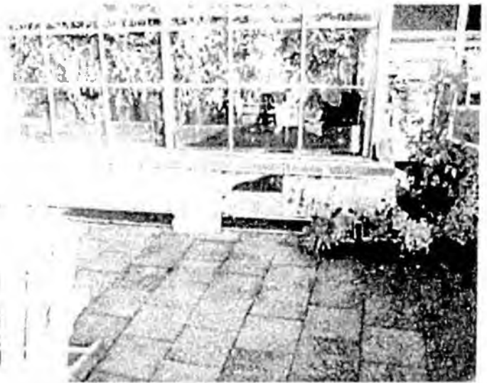
4. Deteriorated siding on wall area below greenhouse structure, Leak #1 is several feet to left of this area
