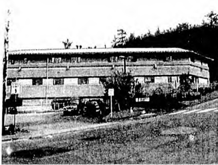
Priority 3 : Ketchikan Pioneer Home Exterior Paint and Repair ($140,590)
