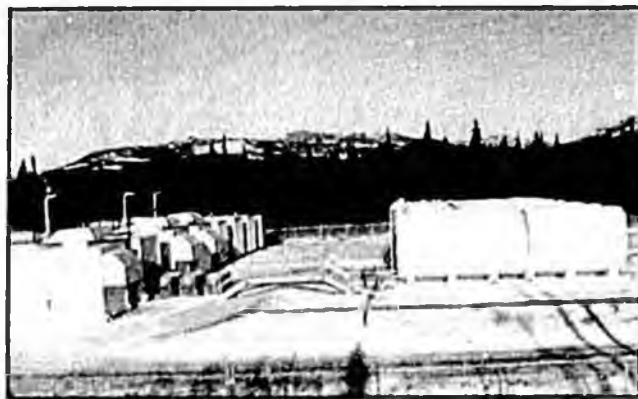
Kalskag's new power plant and bulk fuel tank farm.
