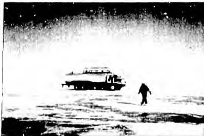
Figure 4: Ice road construction begins when the active layer is satisfactorily frozen. Snow is packed and then pumped water is sprayed onto the snow surface until a sufficient road thickness is attained (photo — W. Morris).
